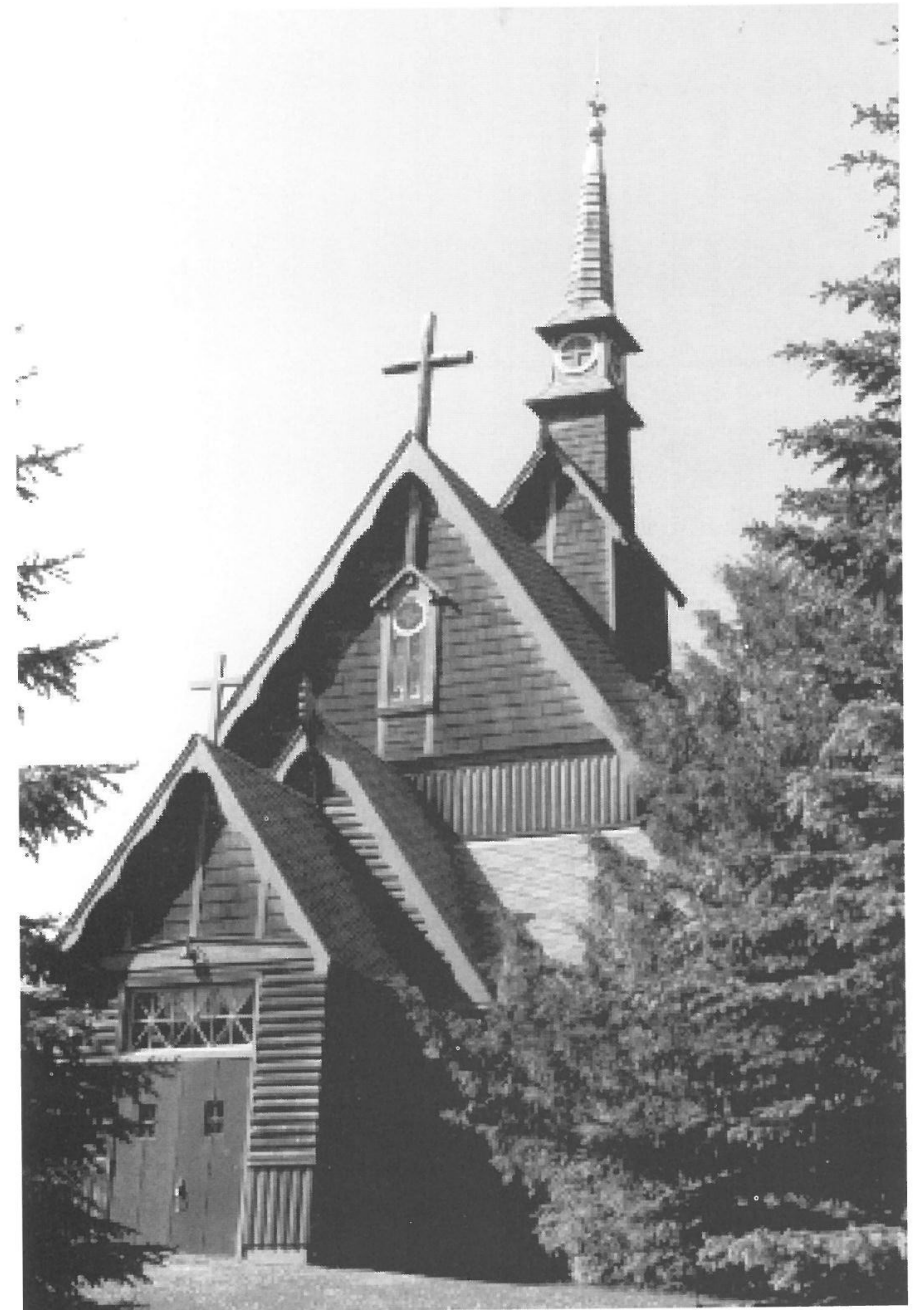
The chapel at Green Lake Bible Camp was patterned after Borgund Stave Church near Bergen, Norway. The chapel was built in 1939-40.
